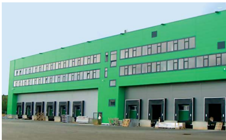
Contemporary logistics facilities in Volozhin
